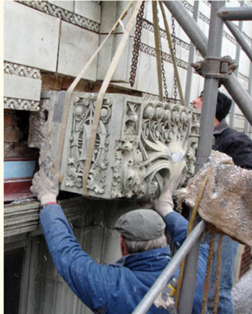
Repaired terra cotta ornamentation is hoisted into place
